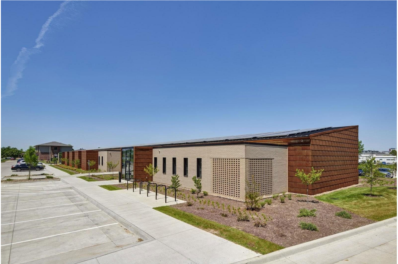
Figure 40. The Guidelink Center, Johnson County, IA
